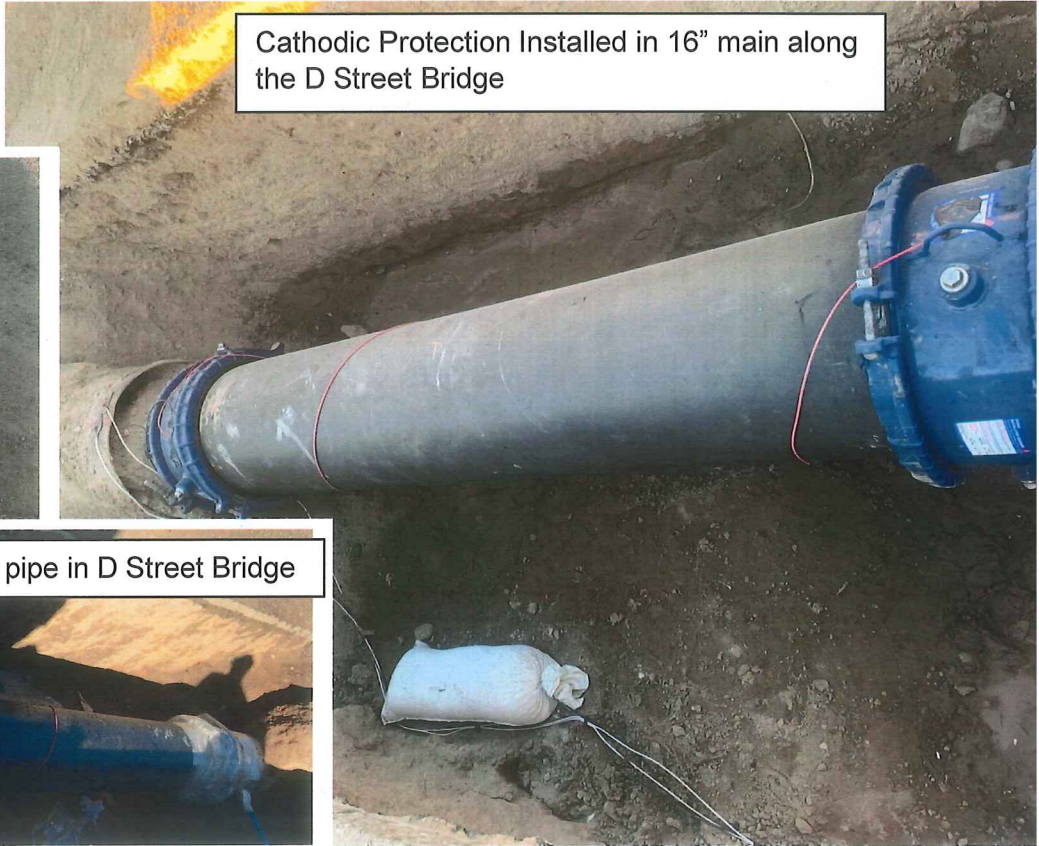
Cathodic Protection Testing Port Installed along on D Street Bridge
